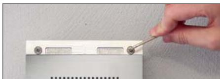
**3** Connect the Intercom station and attach it in the provided on-wall/flush mounting housing, cavity or Behnke column (series 5 only). Re-attach the stainless steel strips in Series 10 devices.
